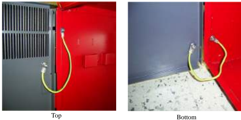
Figure 5-3. Dead front grounding straps
